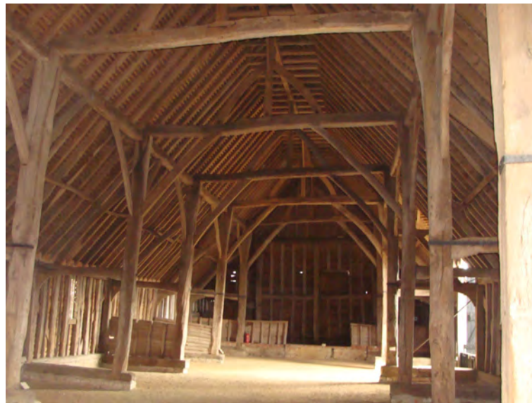
Picture 1.8 Priors Hall barn of mid 14th century origin. It is estimated about 400 oak trees were required for its construction
