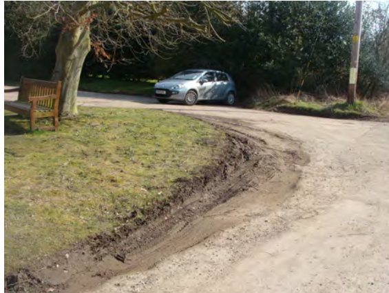
Picture 1.24 Small green near church whose edges are badly eroded by vehicles
